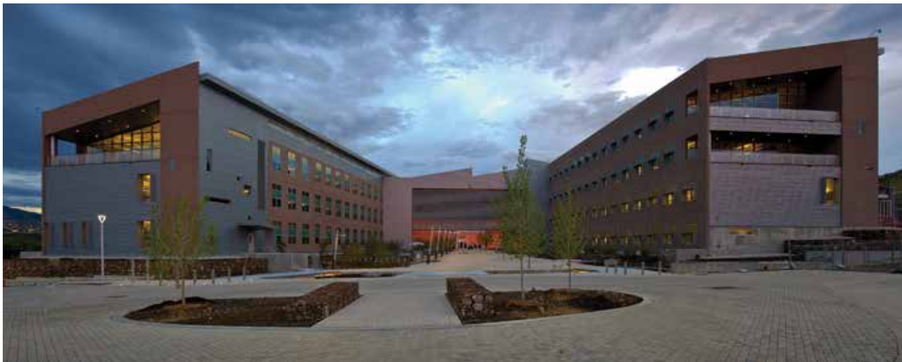
Rocky Mountain Prestress teamed with Thermomass to provide durable insulated panels to protect the NREL Research Support Facility from all manner of Colorado weather while also forming an integral piece of the building's passive heating and cooling operations.
