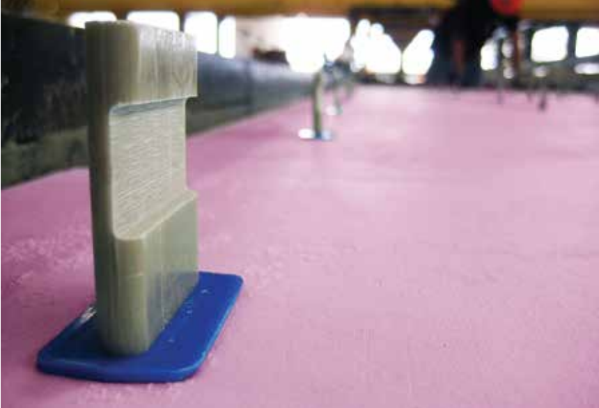
Comprised of fiber composite connectors and prefabricated rigid insulation, Thermomass insulation systems are fully tested, install easily, and have been used in a wide variety of award-winning precast projects.
