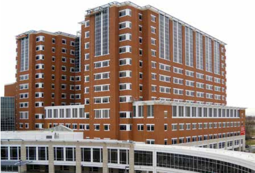
Gate Precast teamed with Thermomass to provide insulated architectural precast cladding panels for the Chandler Hospital Pavilion at the University of Kentucky.
